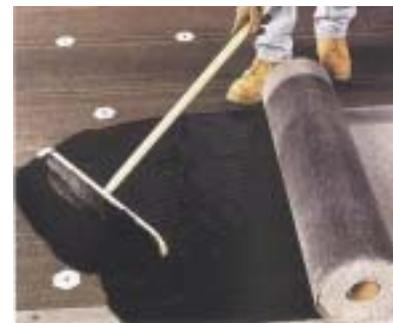
SBS is a high molecular weight polymer that has both thermoset and thermoplastic properties. It gives rubber-like qualities to asphalt roofing membranes and is mopped down with a layer of hot asphalt.
