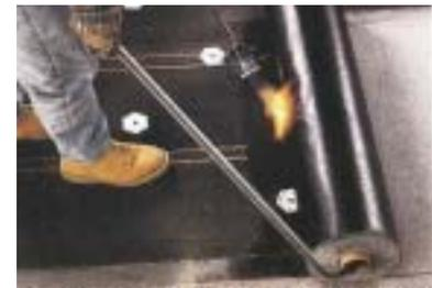
APP is a group of high molecular weight polymer membranes applied to roofs using an open torch.
